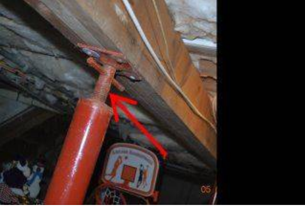
Photo 22-1 use of temporary support columns
